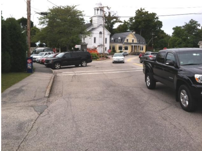
On-street Parking Restricts Sight Distance Looking Left
