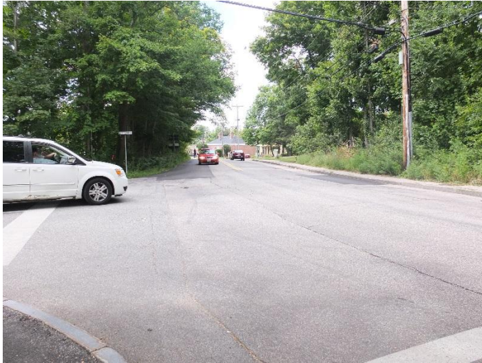
Location of stop bar combined with existing vegetation along south side of Long Sands Road restricts sight distance
